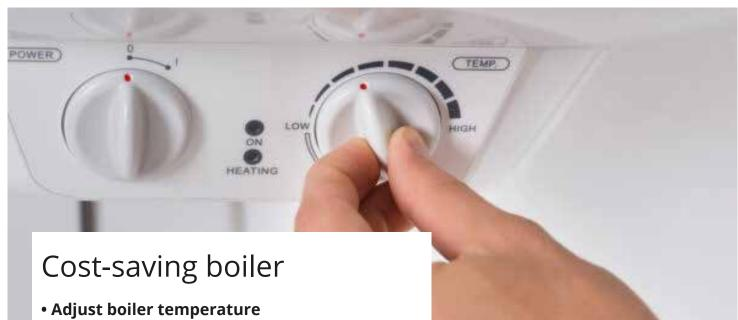
Most boilers have two hot water temperature dials – one for hot water going to taps, and another for hot water going to heating system (if you have heating from boiler). Adjust both dials yourself so they are set at halfway, as 50% boiler heat is enough.
